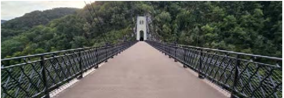
Completed steel decking with sandblasted resin coating and round head bolts
