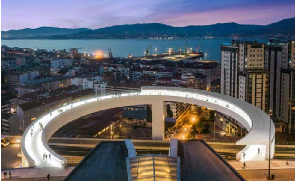
Halo circular footbridge and elevators, aerial view
