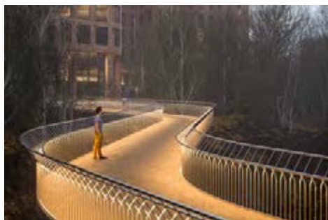
The Cycle Bridge in Stainless Steel
