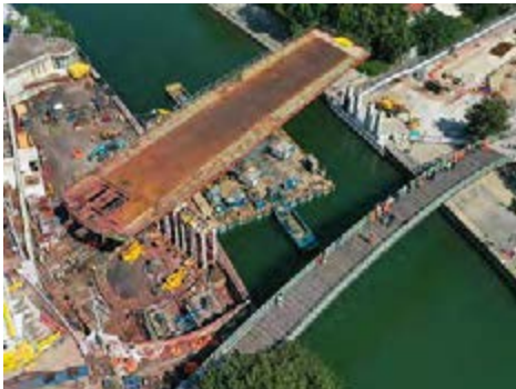
Lucie Bréard footbridge, rotation of the swing bridge © Sernavision/Razel-Bec
