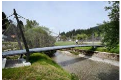
Suspension bridge “Himmelhausmatte- steg”, Trubschachen – Switzerland, span 26 m
