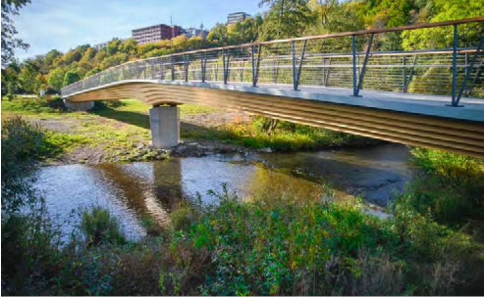
Block girder bridge 'Wehrweide' by Peter Bergmann
