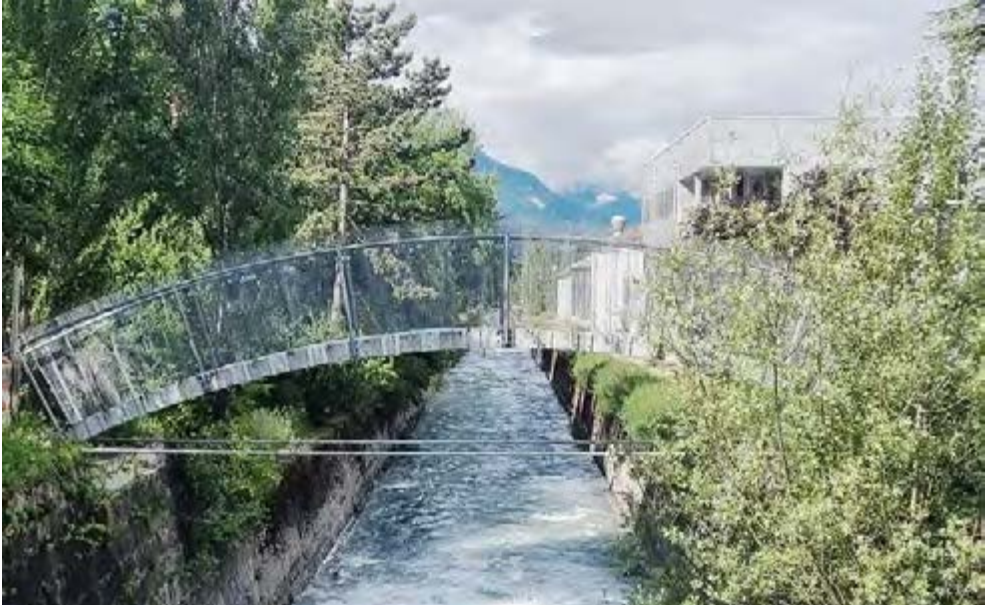
Re:Crete footbridge made of reused cut concrete blocks (© SXL).
