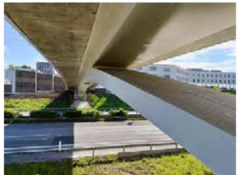
General view of the footbridge from below
