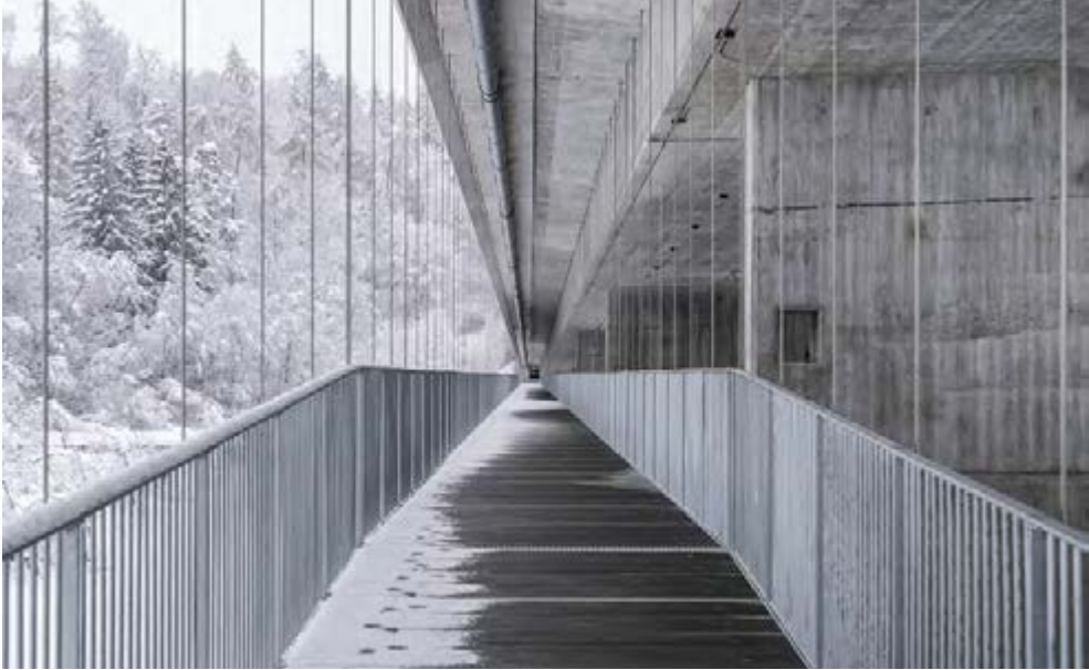
View of the suspended pedestrian bridge “Punetta” along the walking direction
