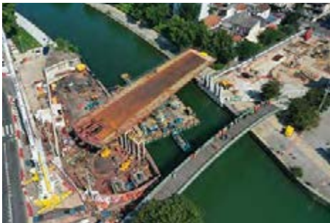
Bridge lifting and rotation © Sernavision/Razel-bec
