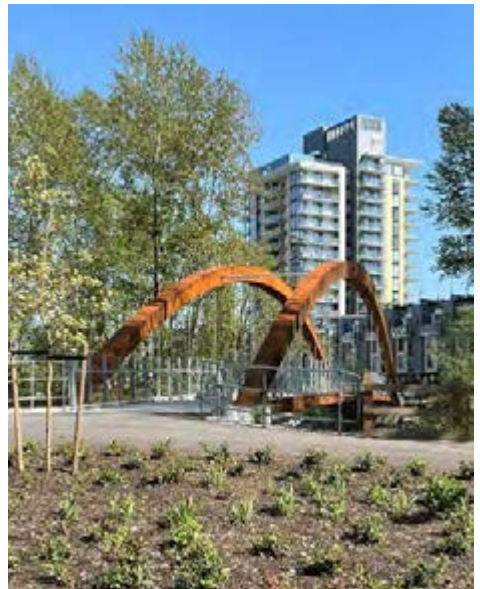
Spirit Trail Lynn Creek Crossing's weathering steel arch nestles below the forest canopy
