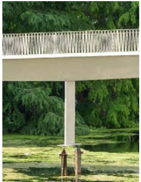
Positioning of the central pier
