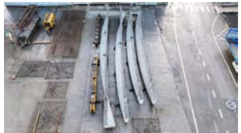
4 precast concrete arches in the factor
