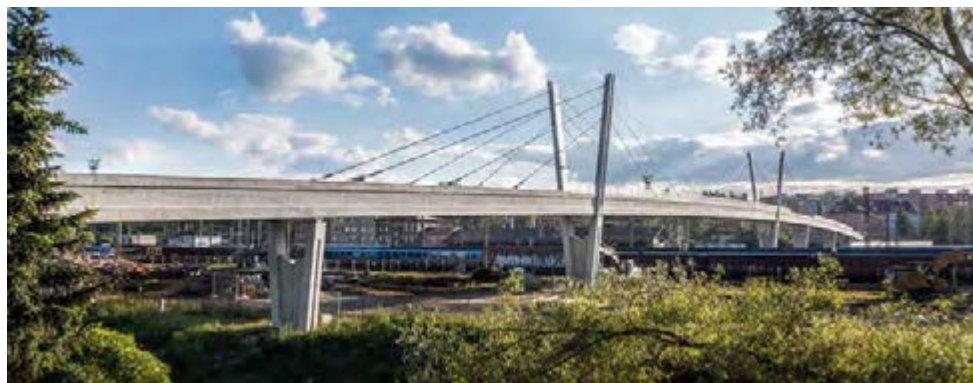
View over central part of footbridge
