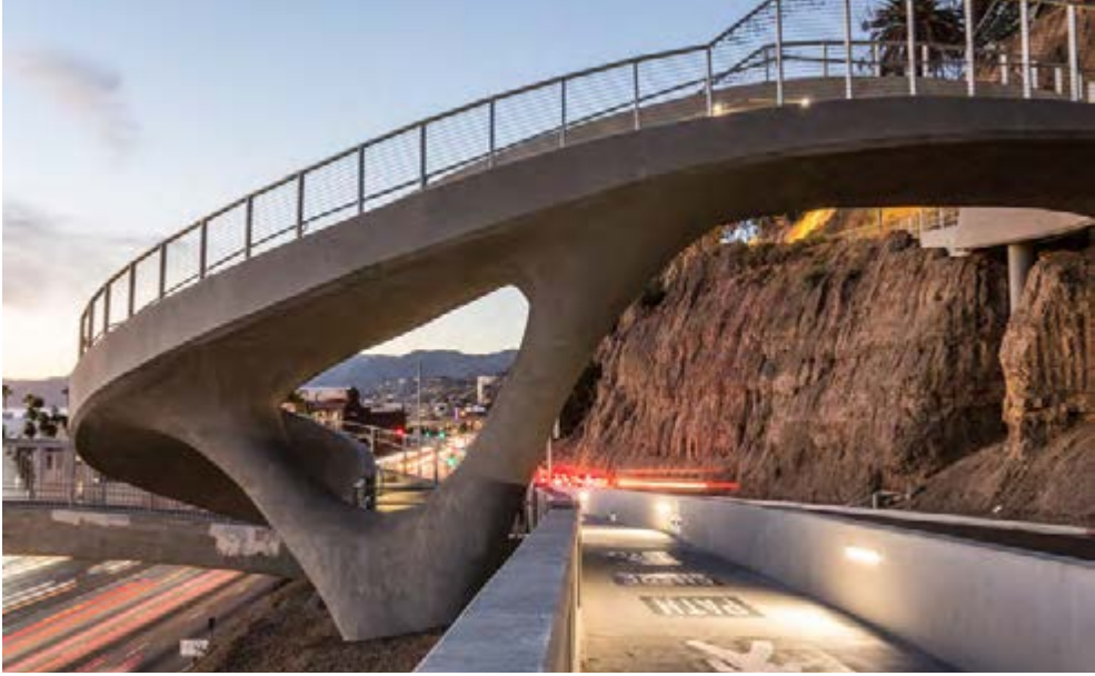
Idaho Avenue Pedestrian Bridge
