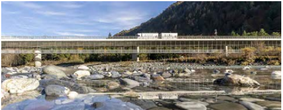
Side view of the bridge “Punetta” attached to the existing highway bridge deck on the upstream side
