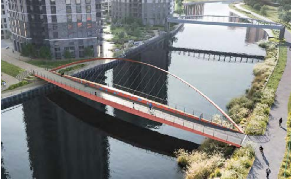
Aerial view of the bridge
