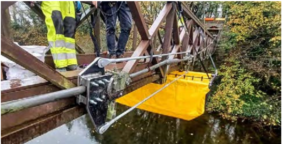
Temporary works in place during construction
