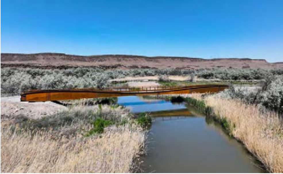
Crab Creek Footbridge
