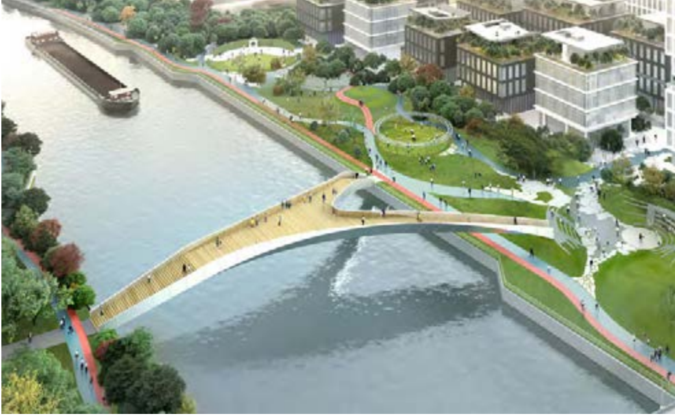
Tianli Bridge. View from the NW
