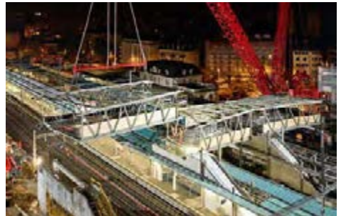
Posing of the third bridge segment; 160 tons at 62 meters
