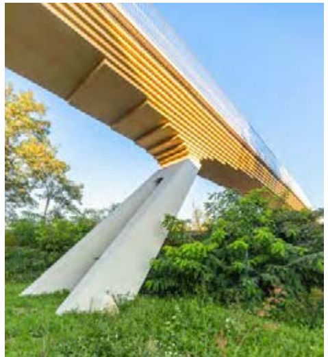
Timber deck and its inclined pier.
