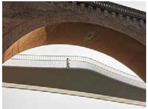
Upstream view of belvedere
