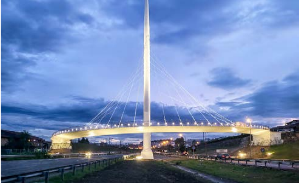
View of the Santullano Bridge with nighttime lighting.
