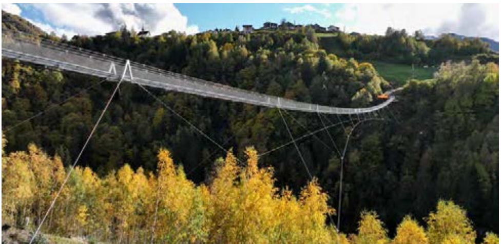
Suspension bridge “LaPendentia”, Disentis – Switzerland, span 270 m
