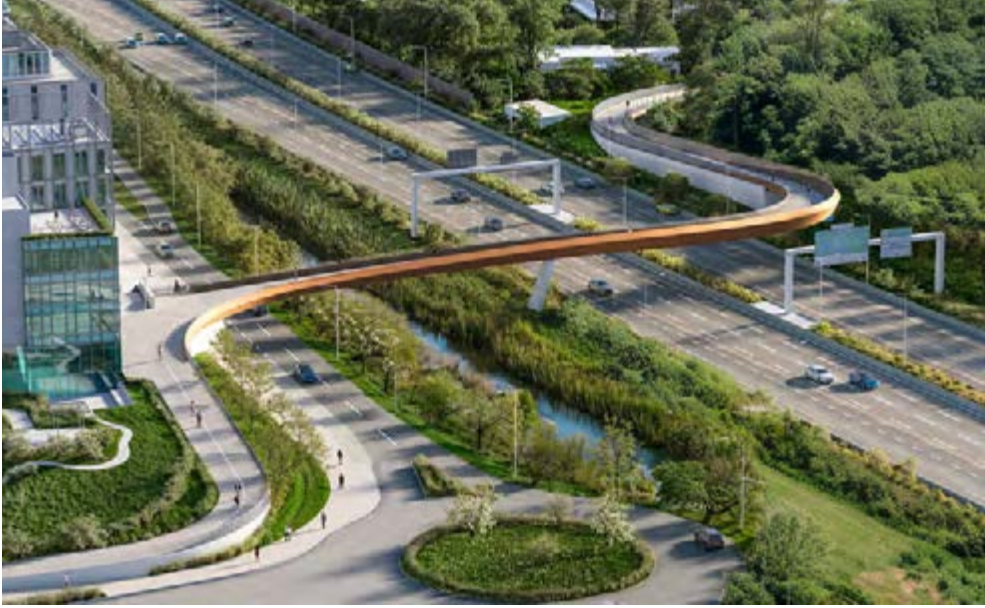
Aerial view of the footbridge
