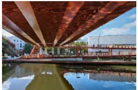
View of the bridge soffit © Michel Denancé
