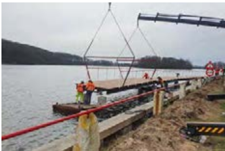
Erection of the bridge elements
