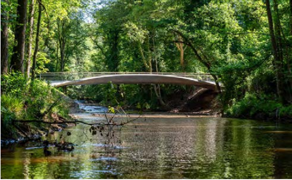
Footbridge with 25.5 m span
