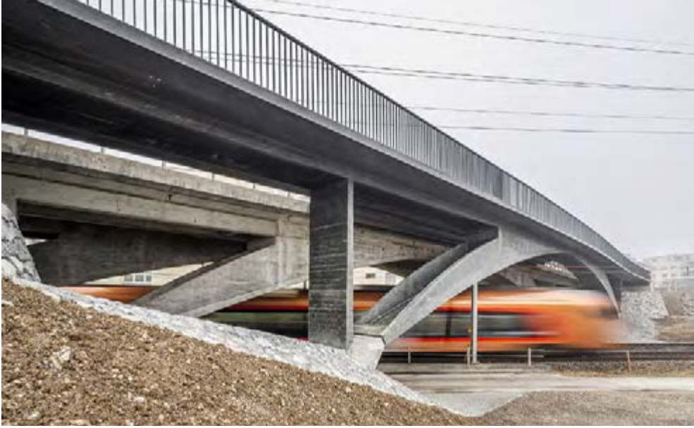
Final state of bridge
