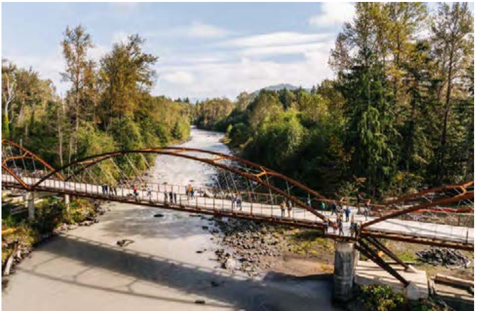
Foothills Trail White River Footbridge
