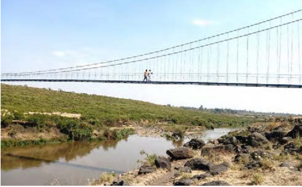
Suspension footbridge over Akaki river, Oromia Ethiopia
