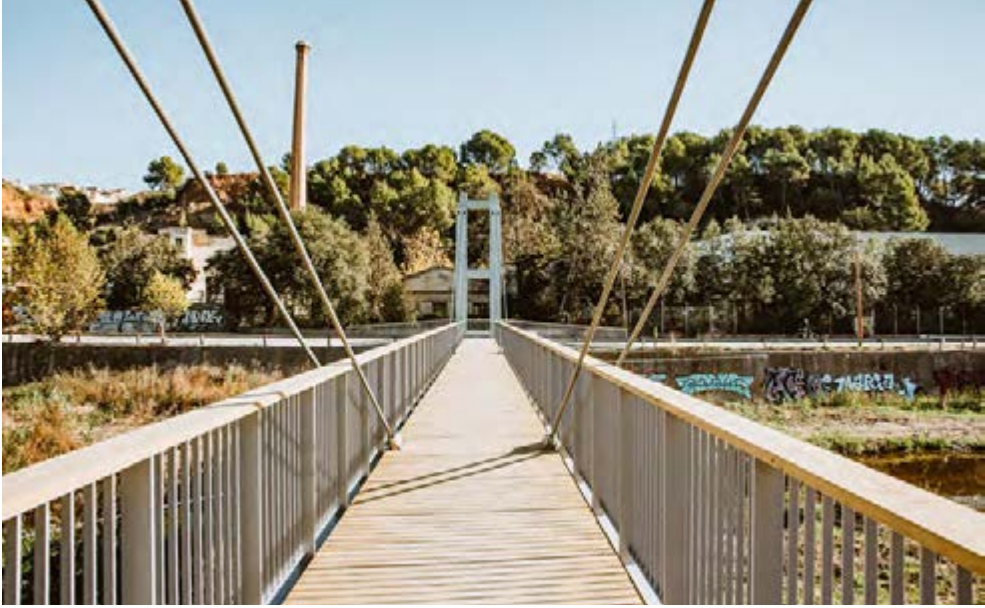
Renovated footbridge over Ripoll River in Sabadell, Spain
