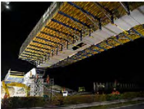
Main span lifting and installation
