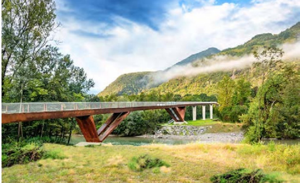
Some general views of the footbridge
