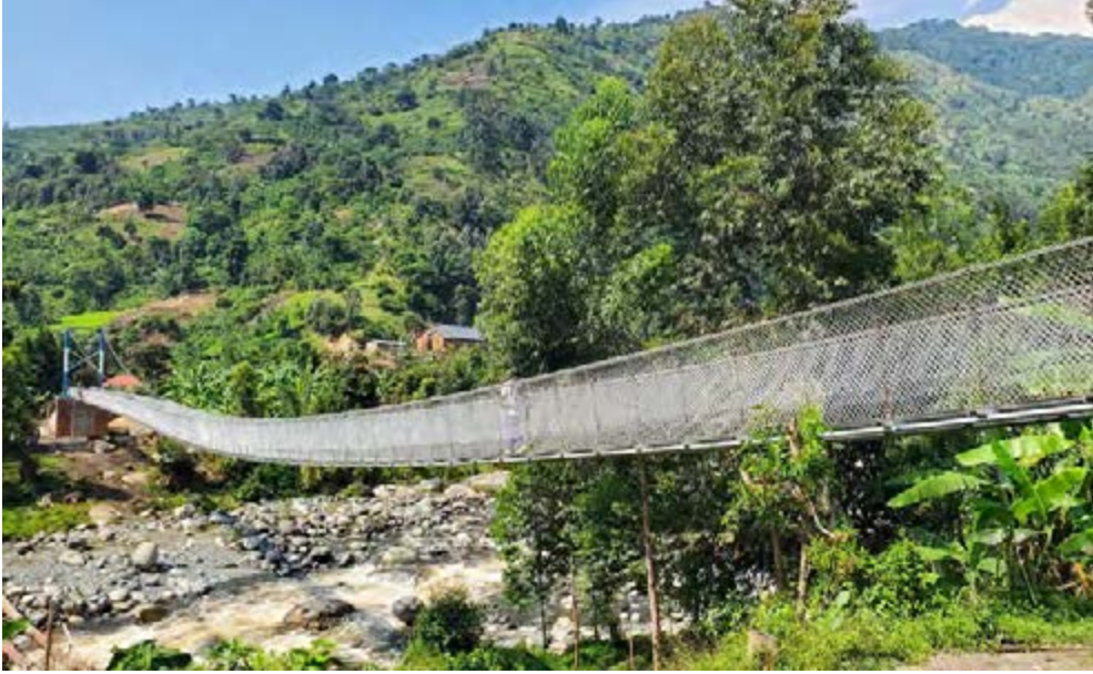
Completed 106 m Hybrid Bridge, Uganda
