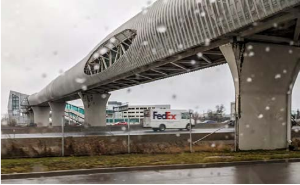
Investigated pedestrian bridge
