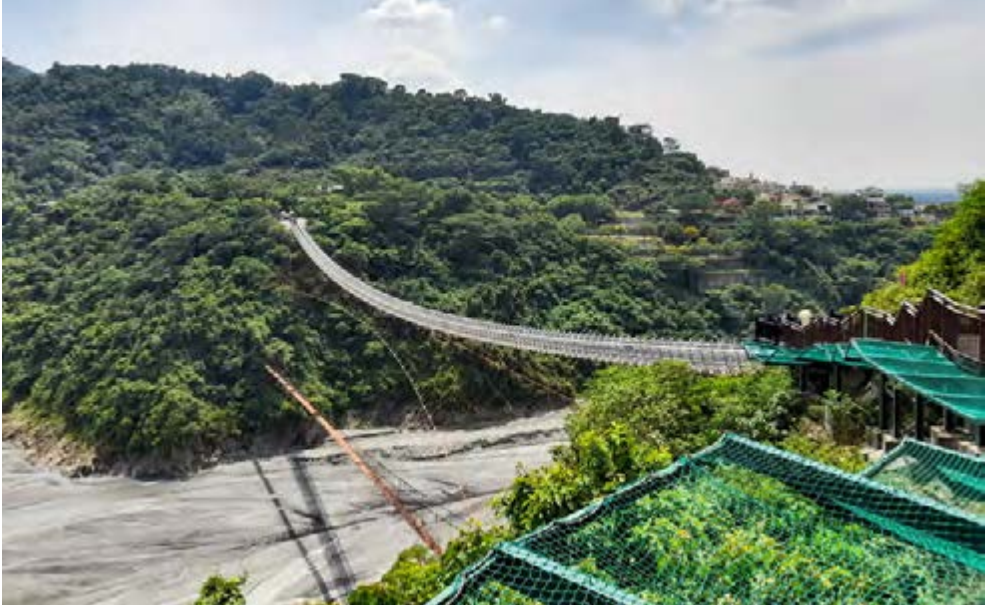
Shanchuan Glass Suspension Bridge
