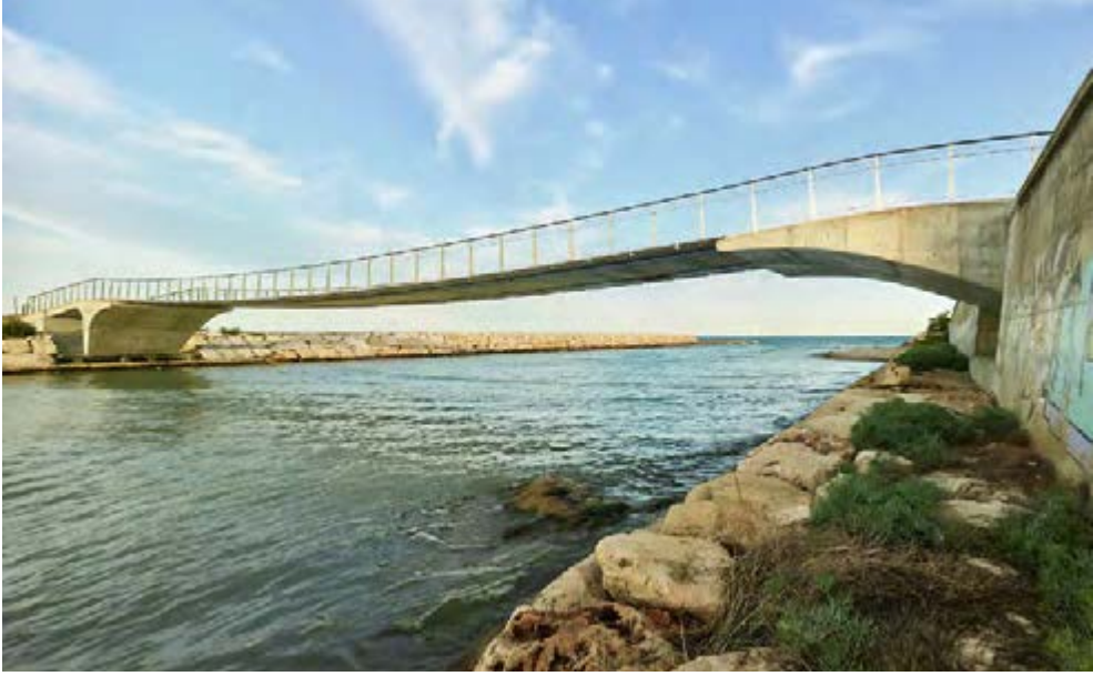
Footbridge in Vinaroz, Spain © Roland Halbe
