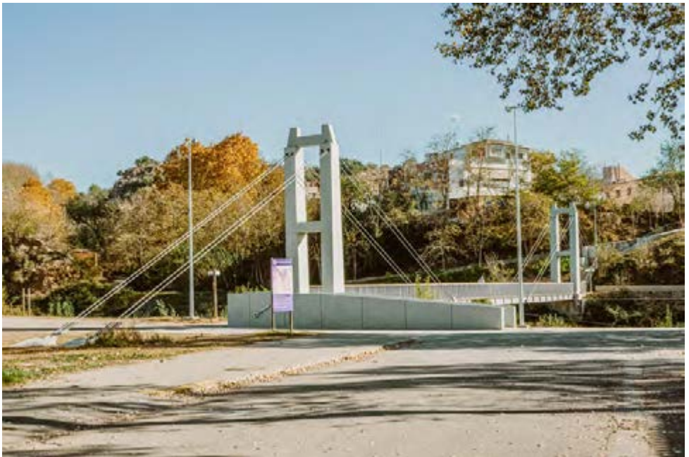
Renovated footbridge over Ripoll River in Sabadell, Spain
